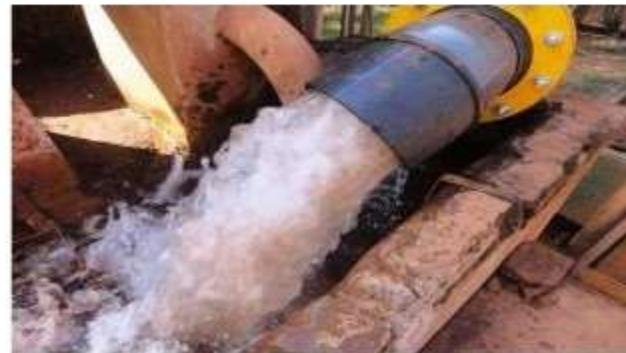
Treated Water from Effluent Treatment Plant being collected in the inlet channel of the Water Treatment Plant for treatment
