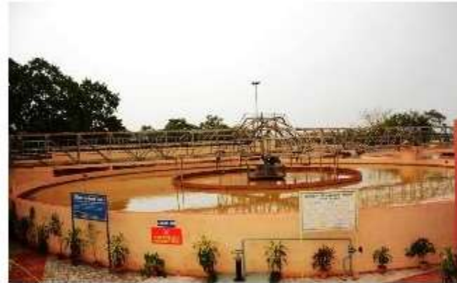
Three Clariflocculators capable of independently treating water @1500 m 3 /hr
