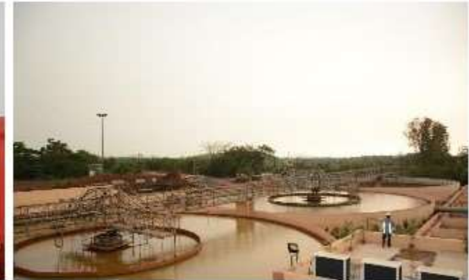
Three Clariflocculators capable of independently treating water @1500 m 3 /hr
