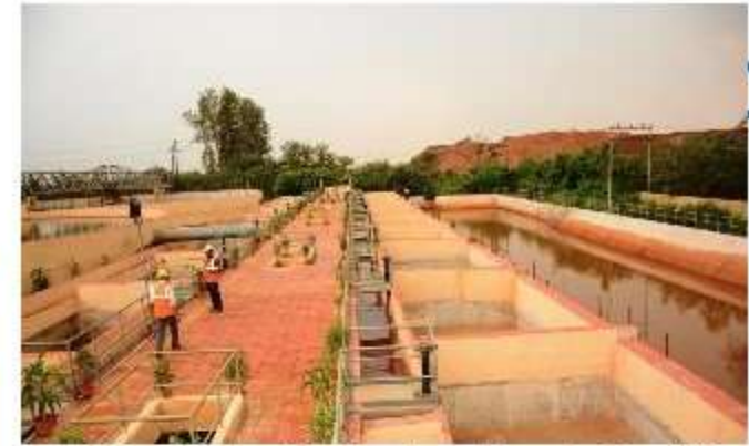
Raw Water Collection Tank and Gravity Sand Filters
